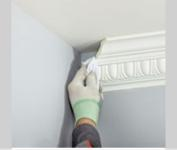
Using the gun, apply a line of adhesive on the whole plane of the article joint, put it on the base surface
