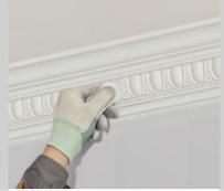
Using the gun, apply a line of adhesive on the whole mounting plane of the article, put it on the base surface
