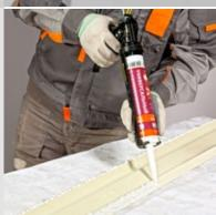
Press with strength and fix for 4-5 seconds
