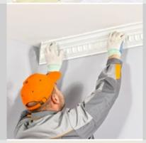
Remove emerged excess adhesive. Complete binding occurs upon expiry of 24 hours
